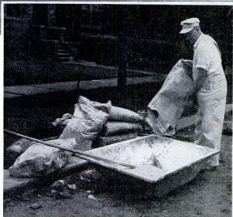
Base-coat plaster comes packaged with aggregate ready-mixed, requiring only addition of water. Reduces chances of error
